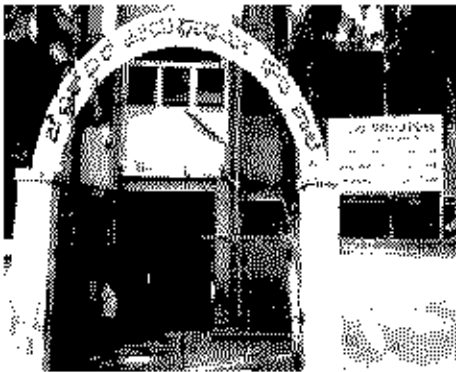
Polling Station Building Front View
