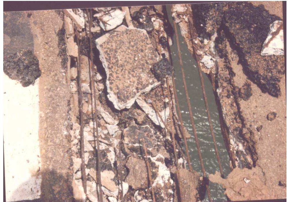
Damage to foot path slab
