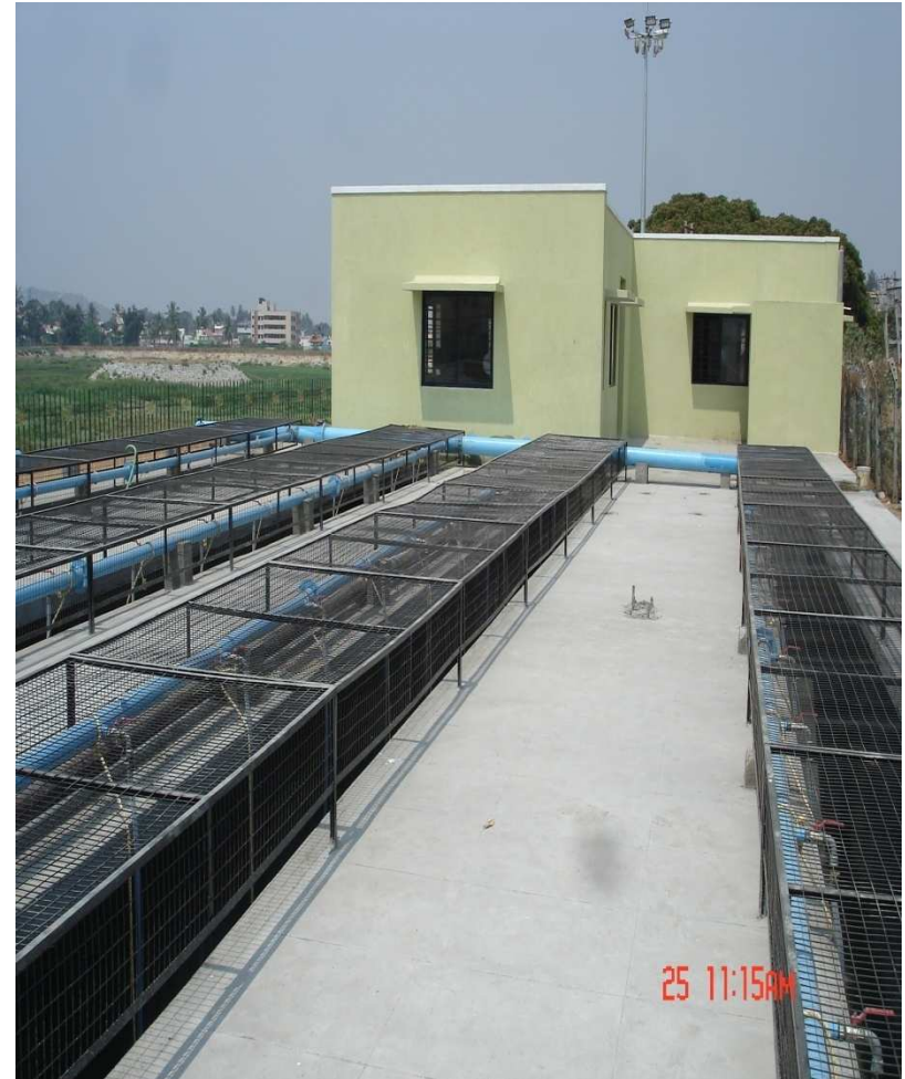
STP Constructed and commissioned
