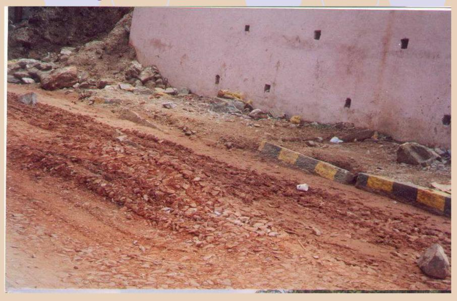
❖ WBM Surface Without Key Aggregates And Excess Binding Material
