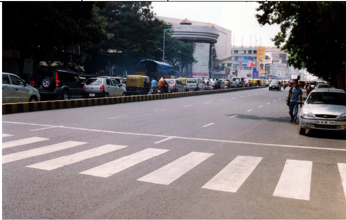
M.G. Road, Completed footpath & Road
