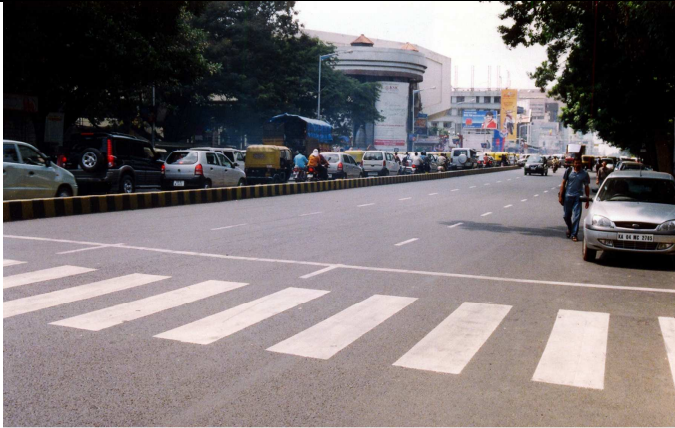
M.G. Road, Completed footpath & Road
