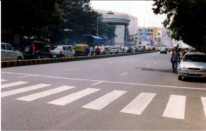
M.G. Road, Completed footpath & Road
